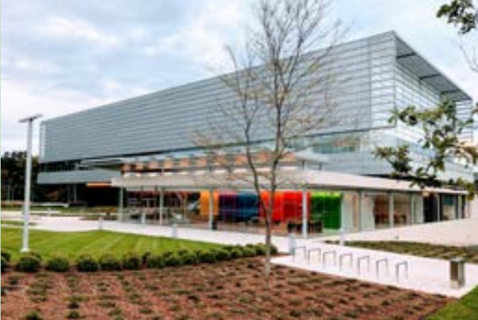
Innovation Partnership Building University of Connecticut Campus 159 Discovery Drive Storrs, Connecticut 06269
